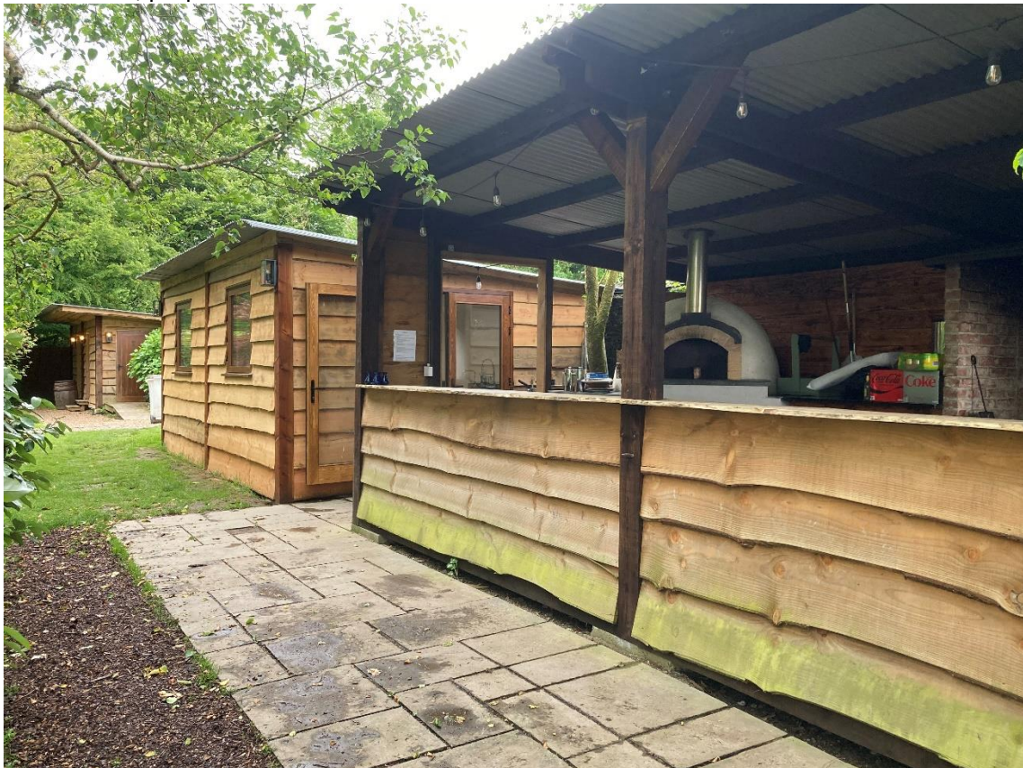
Fire kitchen, prep kitchen and toilet block
